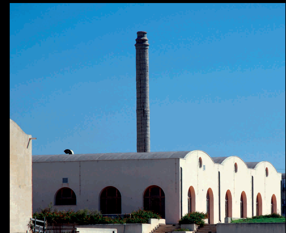
Granitola, tonnara - tuna warehouse
